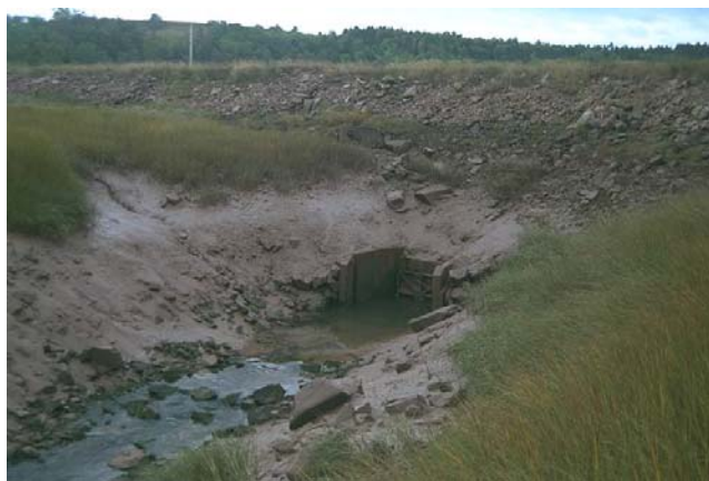
Figure 11. A wooden aboiteau (one way drainage valve) in a dyke near Delhaven.
